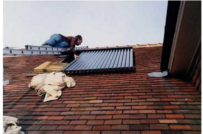
The Greenhouse has two sets of 30 'Thermomax' evacuated tubes each measuring 1.96m by 2.12m with a total surface area of collector tubes of 7.8m<sup>2</sup>.
