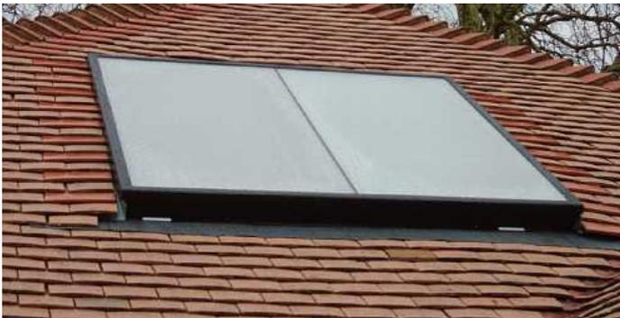
*Flat plate collectors comprise an absorber plate with a transparent cover to collect the sun's heat. Hot water systems that have flat plate collectors on the roof have an efficiency of around 30-35%.*
