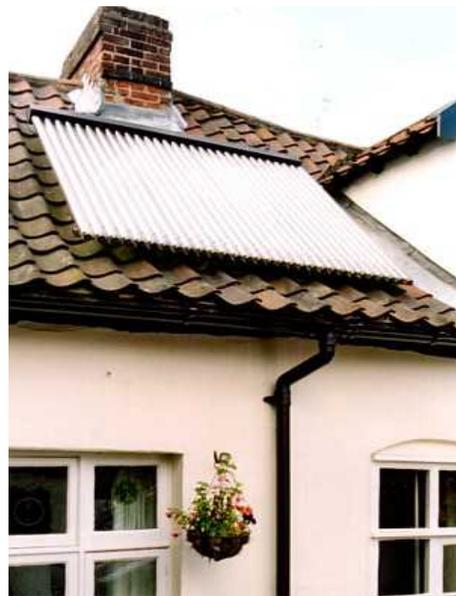
*Evacuated tube systems comprise parallel rows of evacuated tubes. Heat is prevented from escaping by a partial vacuum surrounding the tubes, providing better performance in the winter months. Hot water systems that use evacuated tubes occupy a smaller area and have a efficiency of around 35-40%, but are generally more expensive.*
