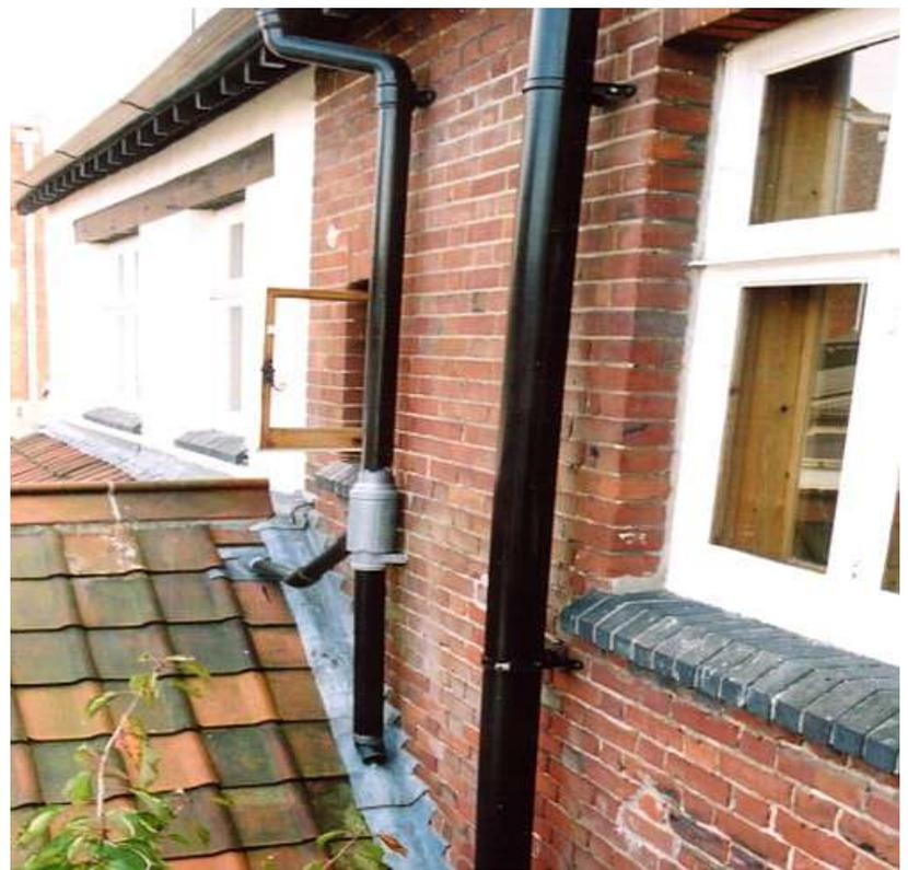
'Wisy' (filter) directs rainwater to the storage tank. The filter can be maintained easily via a 1st floor window.
