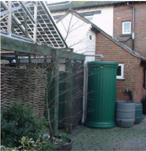
To date the rainwater collection system at the Greenhouse has captured over 297 cubic metres of rainwater (approximately 100 cubic metres per year). This is around 40% of the total volume of water used in this busy public building. It is estimated that a further 50 cubic metres is collected and used on the garden per year.
