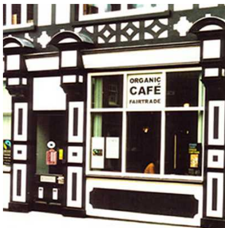
Auro external wood paints were used on this highly decorative building.
