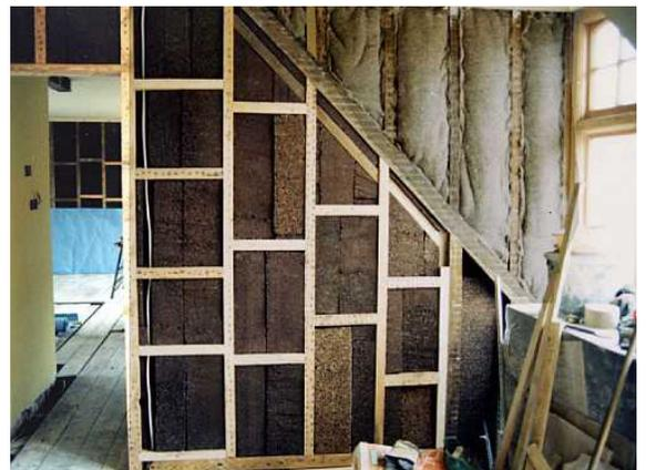
*Wool used in the dormers on the top floor (top right hand-triangle). Cork used in all wall and partition areas.*
