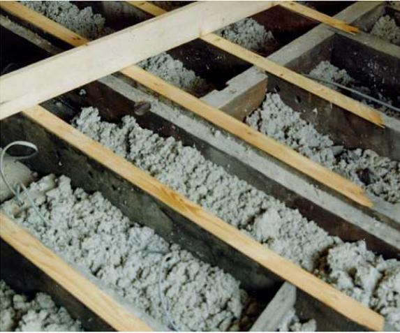
*Recycled paper used for all floor/ceilings to provide sound and heat insulation.*
