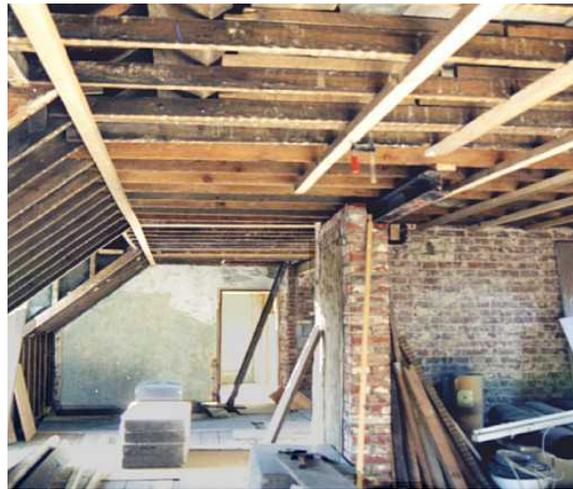
*Crosshatch timbers added to the ceiling of the top floor/roof increased the available depth for recycled paper insulation.*
